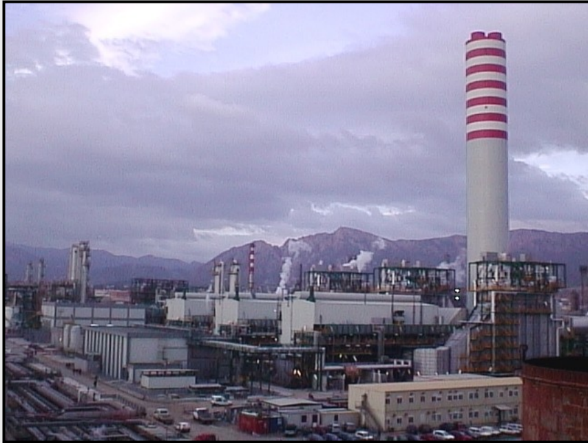
SARLUX IGCC PLANT
