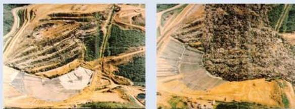
Landfill failure (Kettelmann Hills, 1988)
