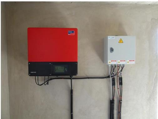
Fig. 3.4: Inverter and DC protections
