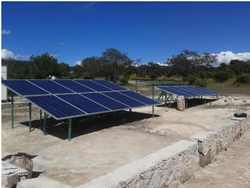
Fig. 3.3: PV modules installed (20 units)
