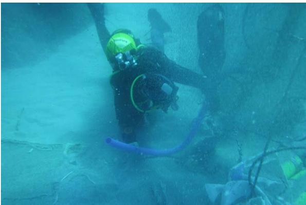
Fig. 2: Excavation of escape-structures at 26 m depth using the newly designed airlift-pump.
