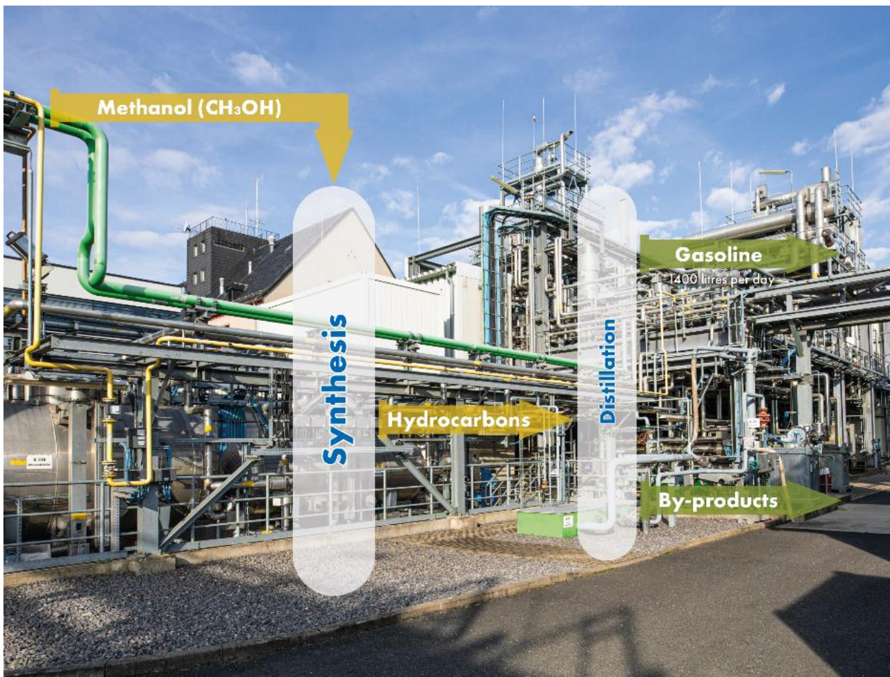
Methanol-to-Gasoline process in the large-scale synthesis test plant
