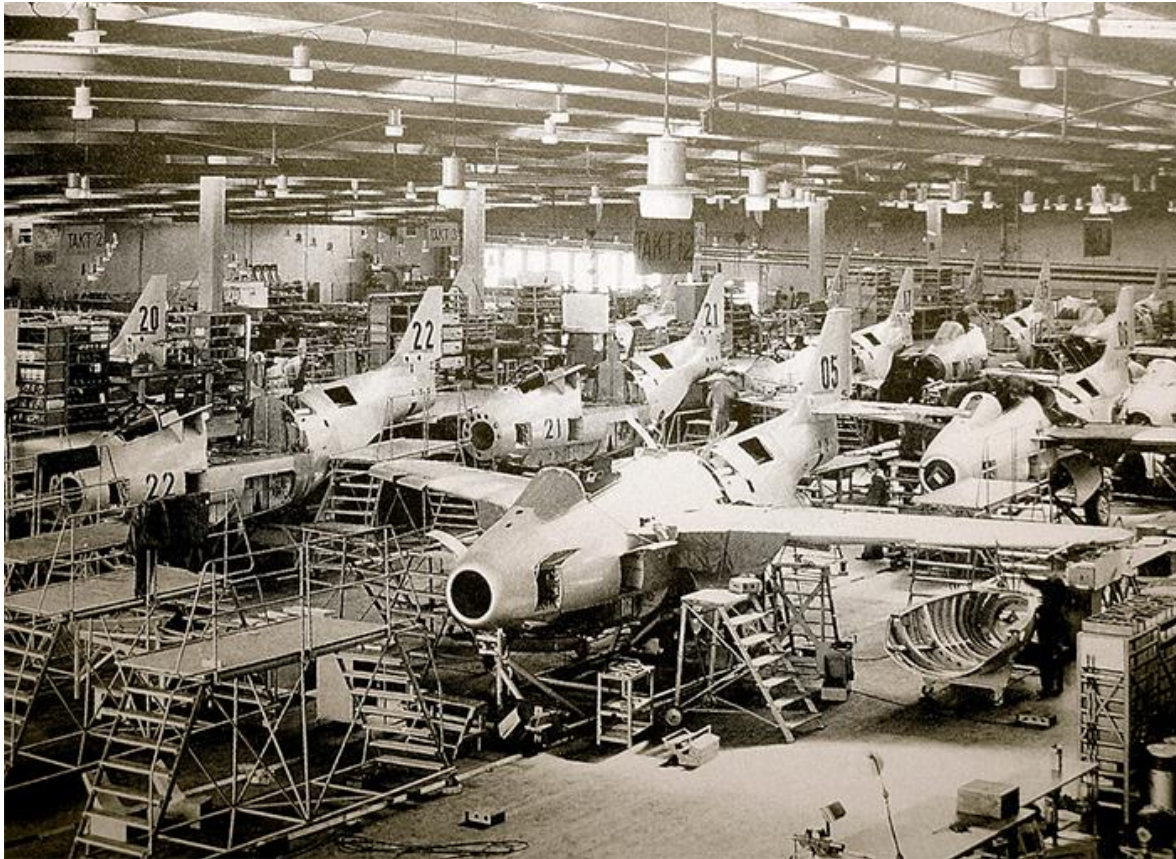
Fig. 7.2: Underground factory SAAB Aircraft (UGE, 2020)
