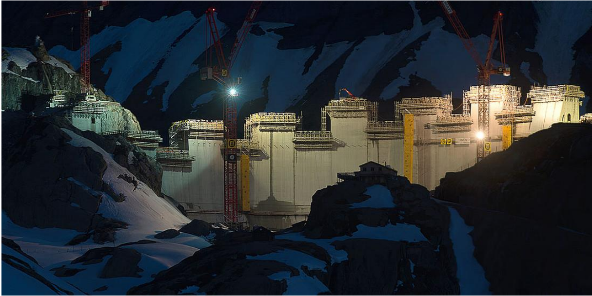
Fig. 2.15: Dam during construction (Nant de Drance HPS, company material)
