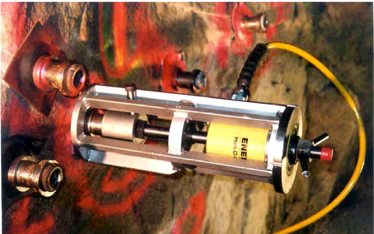
Fig. 6.5: Anchor pull-out test in the field
