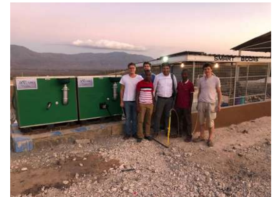
Installation of the Smart Biogas Plants at TTU
