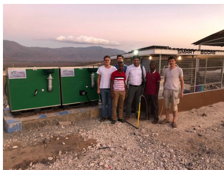
Installation of Smart Biogas Plants at TTU
