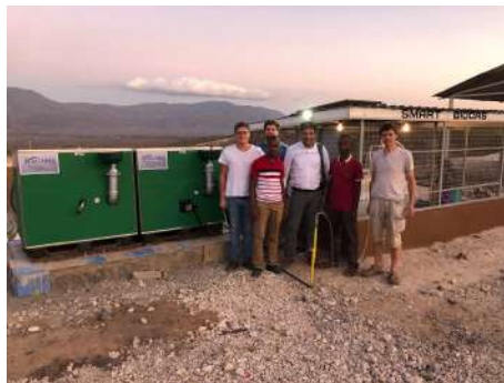
Installation of the Smart Biogas Plants at TTU
