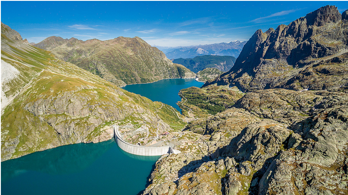
Fig. 2.9: Aerial photo showing the two lakes and the dam (Nant de Drance HPS, company material)
