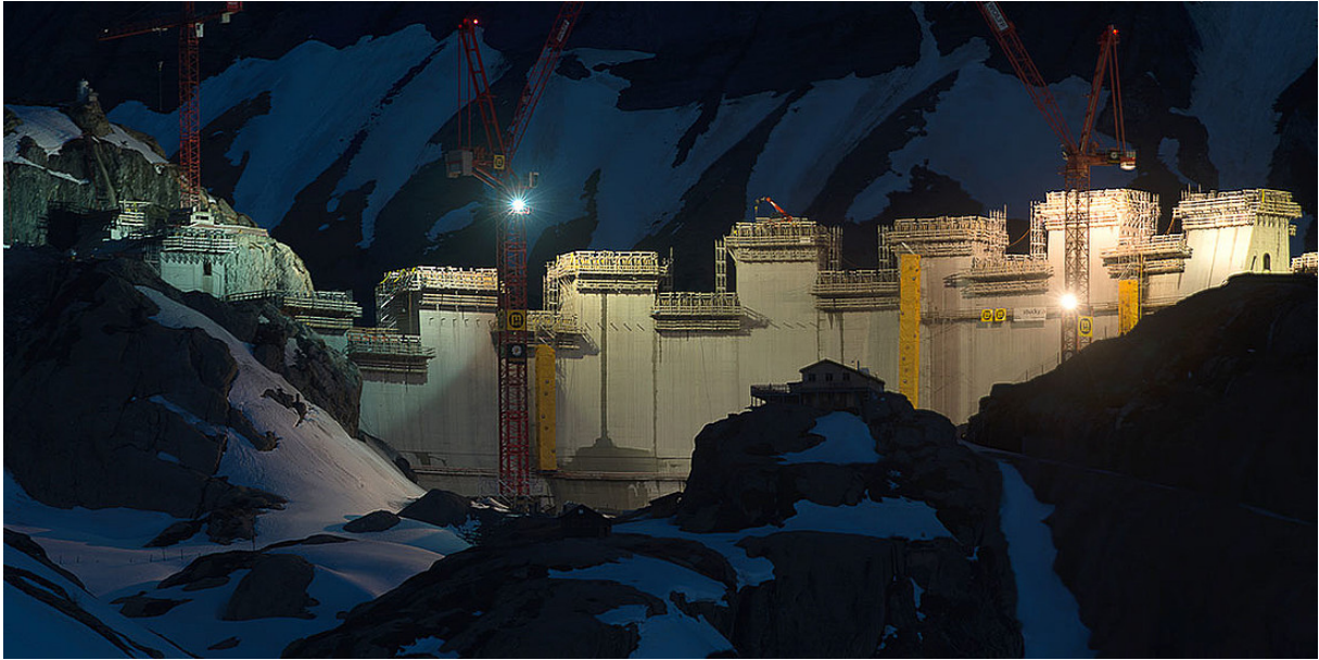
Fig. 2.11: Dam during construction (Nant de Drance HPS, company material)
