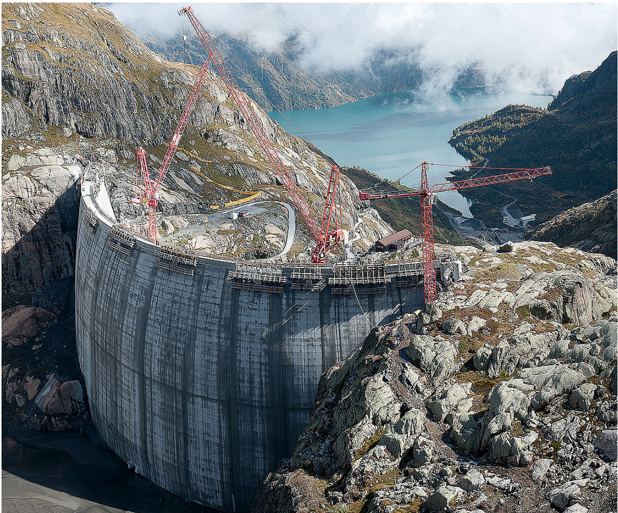
Fig. 2.12: Dam during construction (Nant de Drance HPS, company material)
