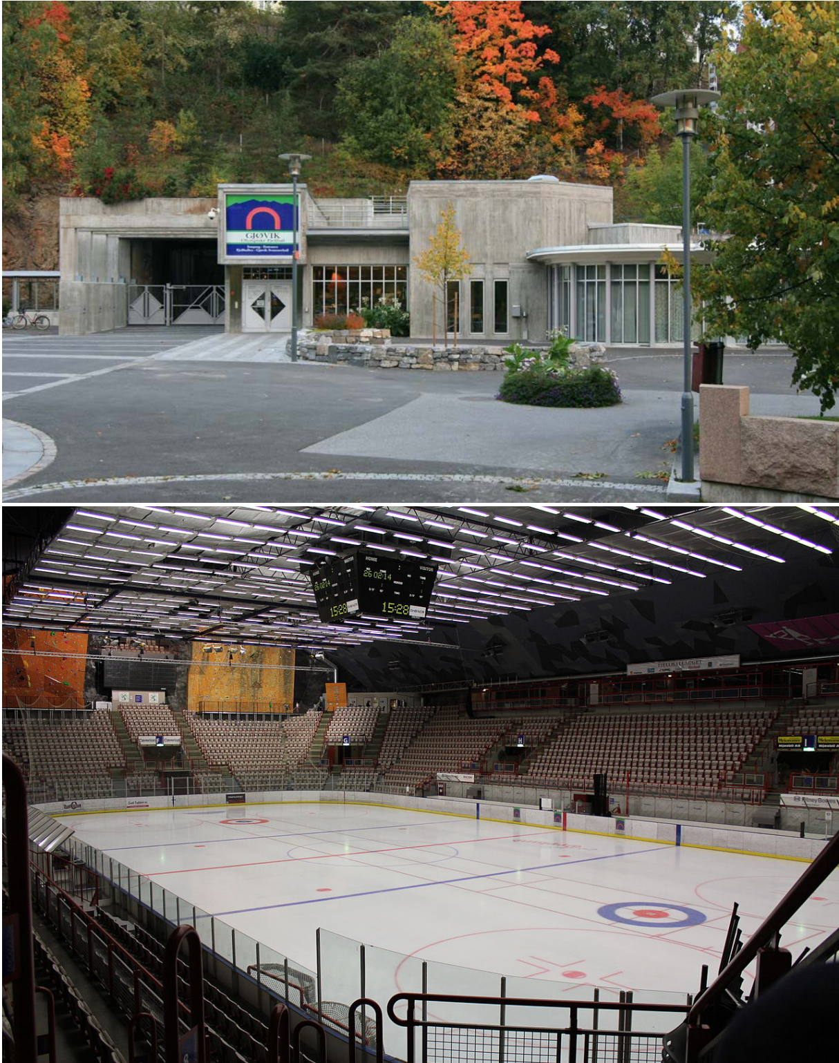
Fig. 8.3: Underground Gjøvik olympic cavern hall, Norway (Holmstad, 2014)
