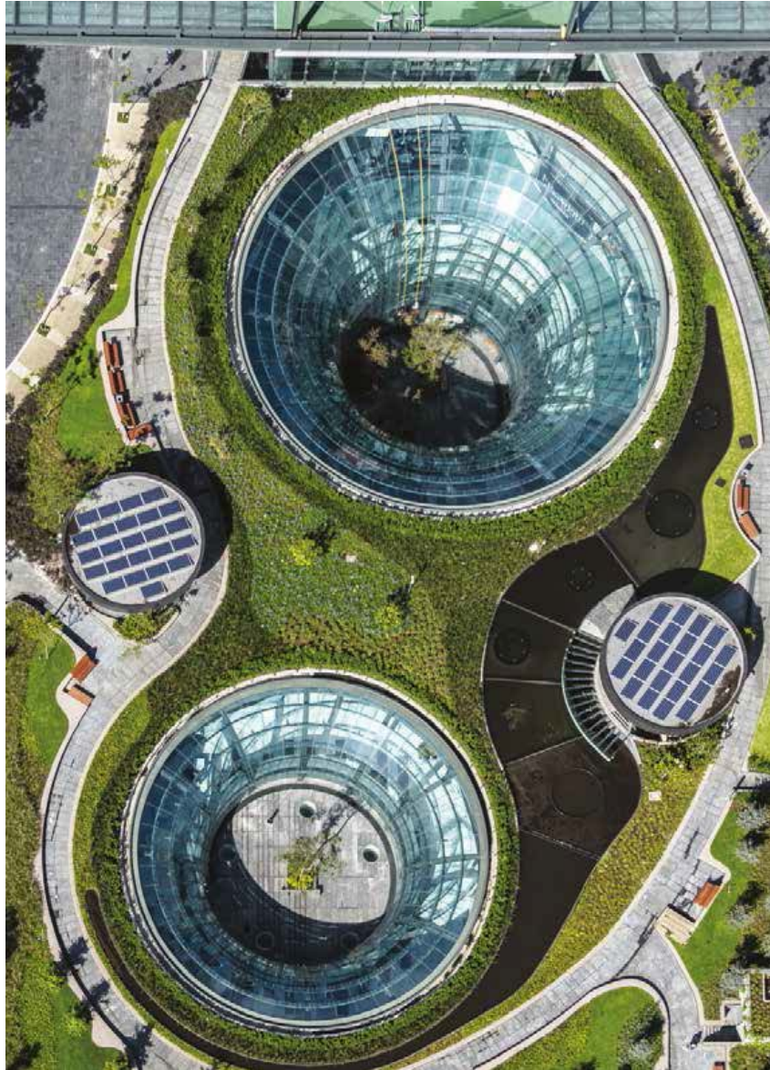
Fig. 8.9: Santa Fe Garden project in Mexico (WSP, 2018)
