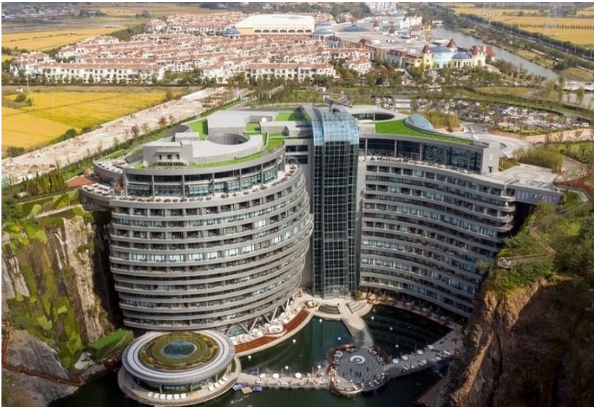
Fig. 8.5: Hotel and congress complex in an old quarry near Shanghai, China.
