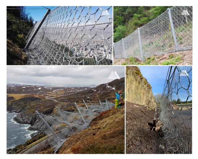
Fig. 4.6: Exemplary: flexible rockfall protection barriers in-situ (company material: Geobrugg)
