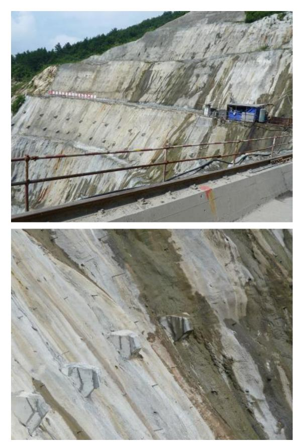
Fig. 3.2: Rock slope stabilised with berms, shotcrete, systematic pre-stressed anchorage and relief boreholes for dewatering (water dam project, China)
