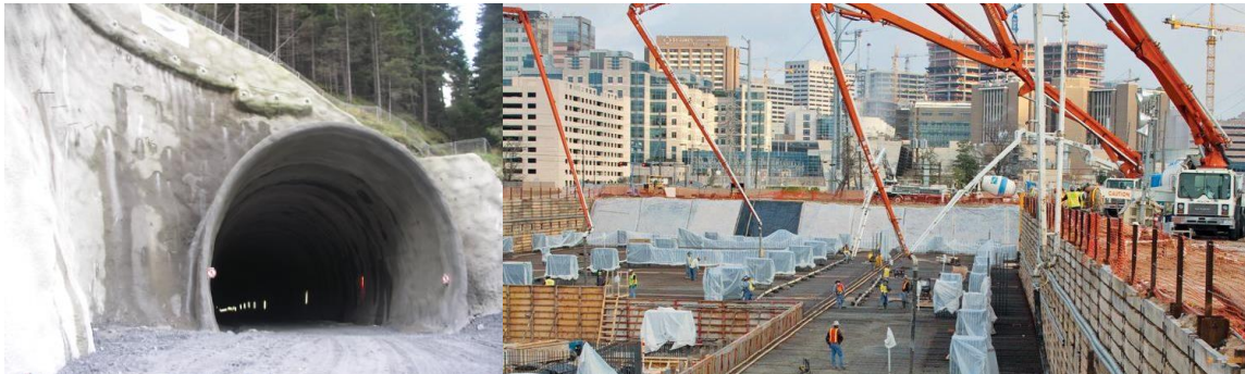
Fig. 1: Flowable concrete applications (left: shotcrete, right: pumped concrete; company material)
