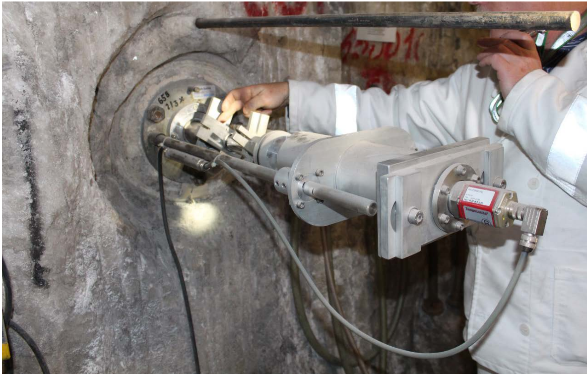
Fig. 4.1.5. Extensometer head (installation in an underground mine)
