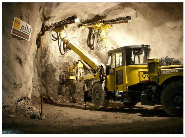
Fig. 20: Drill jumbo in operation (company material)
