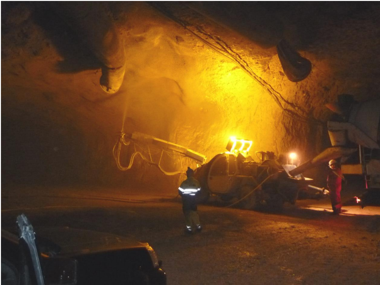
Fig. 7: Application of wet sprayed concrete in a mine
