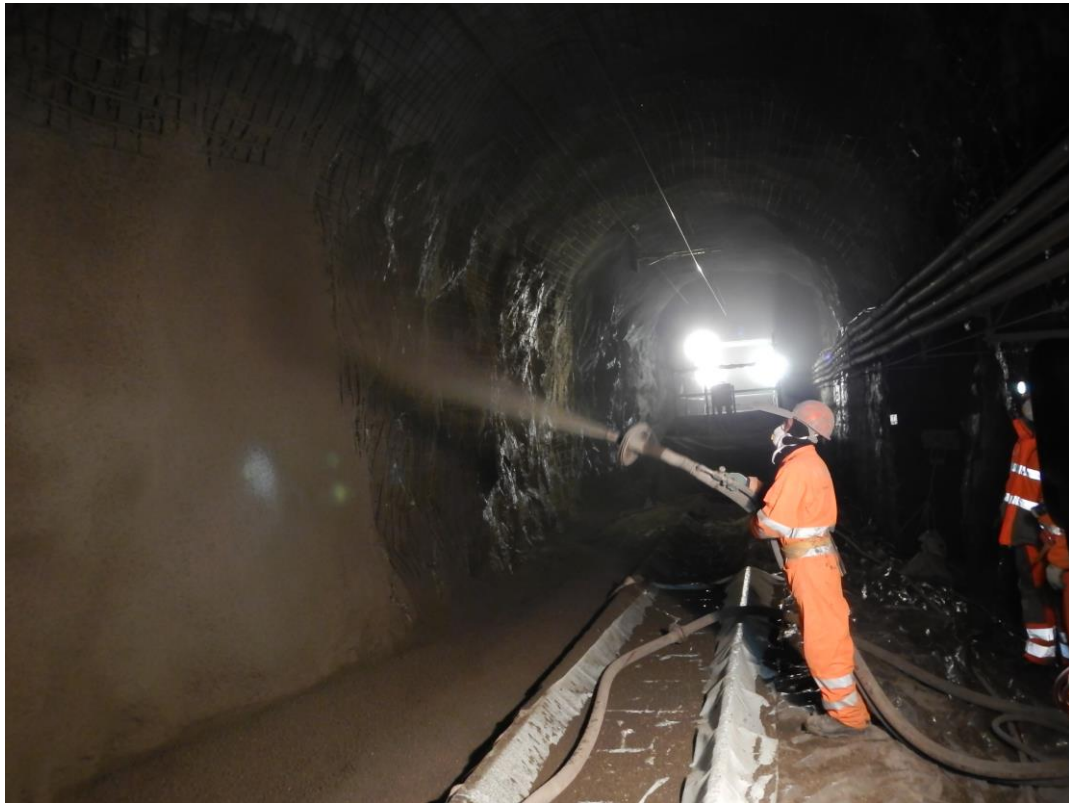
Fig. 5: Application of dry sprayed concrete (I) (Source: AF Toscana AG)
