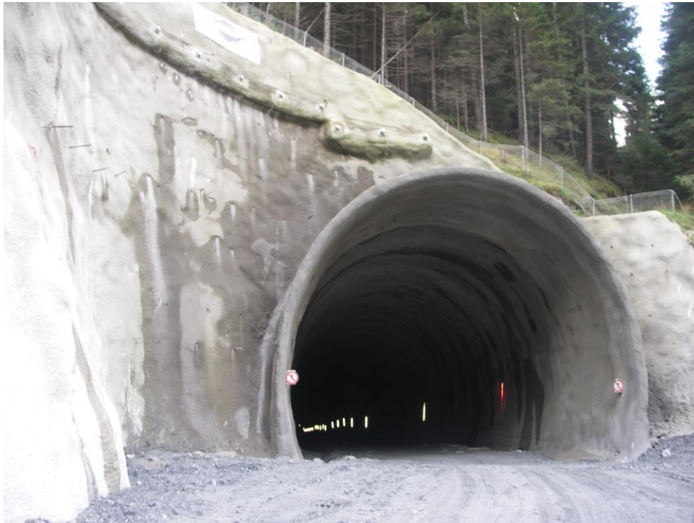
Fig. 2: Shotcrete application at a tunnel portal
