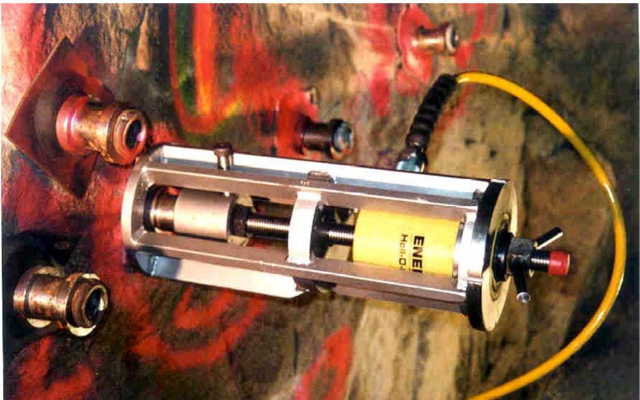
Fig. 6.5: Anchor pull-out test in the field
