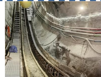
② Tunneling in the downward curve section
