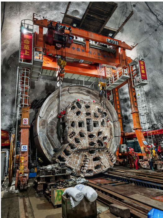
Split disassembly technology for main machine and back-up system in inclined shafts
