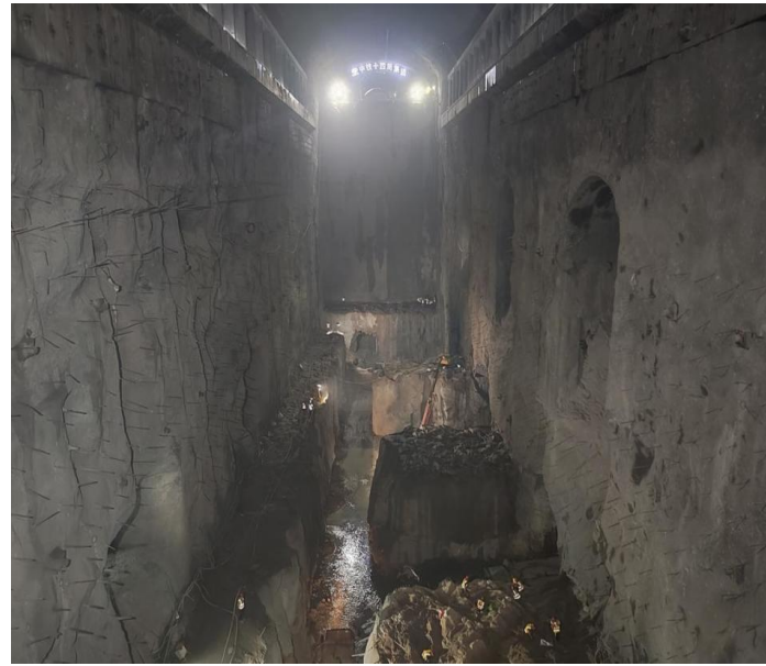
Underground powerhouse and drainage tunnels
