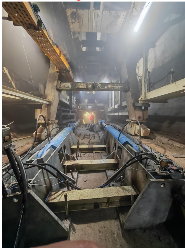
External cylinder + winch-assisted traction disassembly technology
