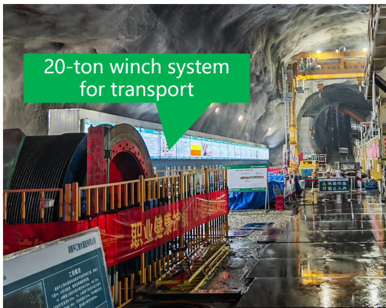
Winch wire rope traction system technology adaptable to vertical curves
