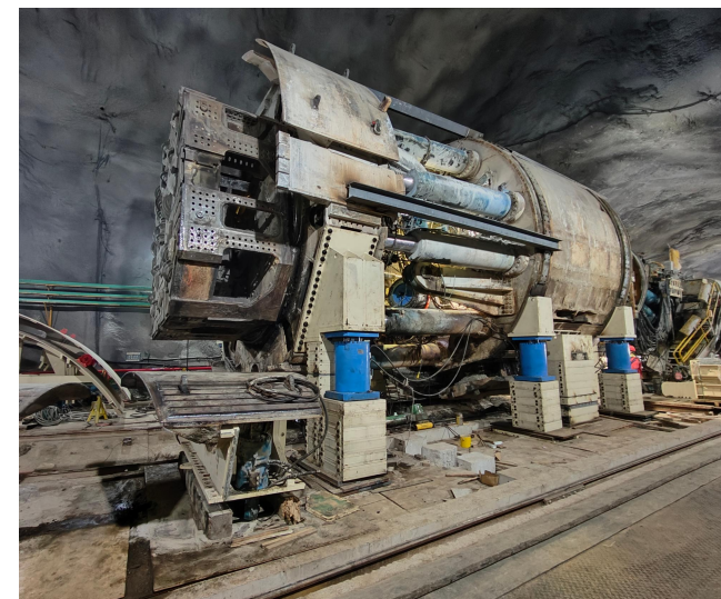
TBM synchronous jacking and diameter changing technology
