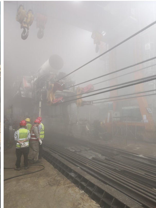
External cylinder + winch-assisted traction disassembly technology
