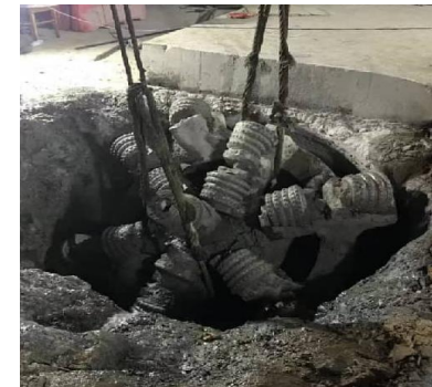
Directional drilling + raise boring + drill-and-blast reaming process
