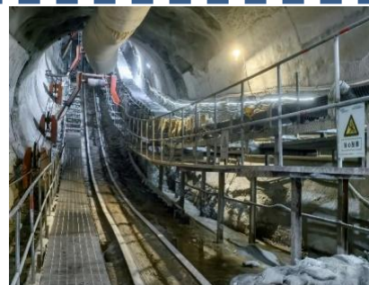
① Launch to the bottom of the inclined shaft
