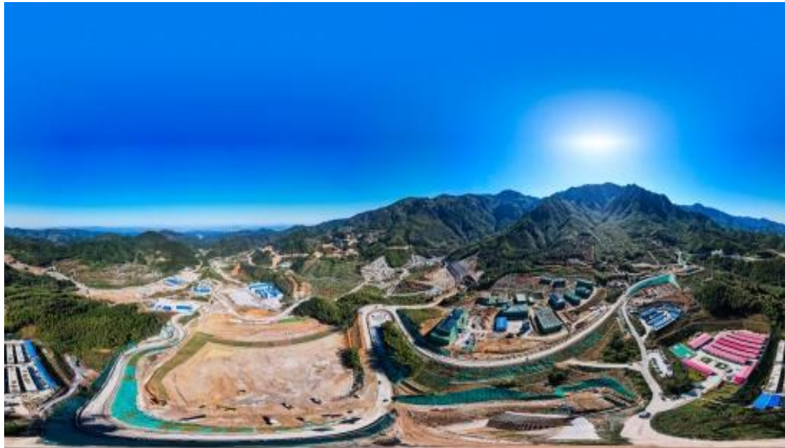
Pumped Storage Power Stations
