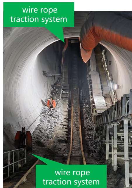
Winch wire rope traction system technology adaptable to vertical curves
