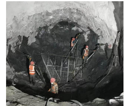
Directional drilling + raise boring + drill-and-blast reaming process
