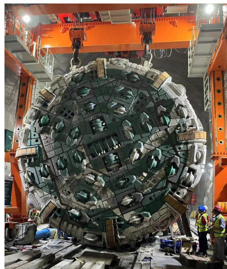
Hydraulic jack-up gantry crane
