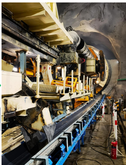
Horizontal tunnel assembly and turning launch technology
