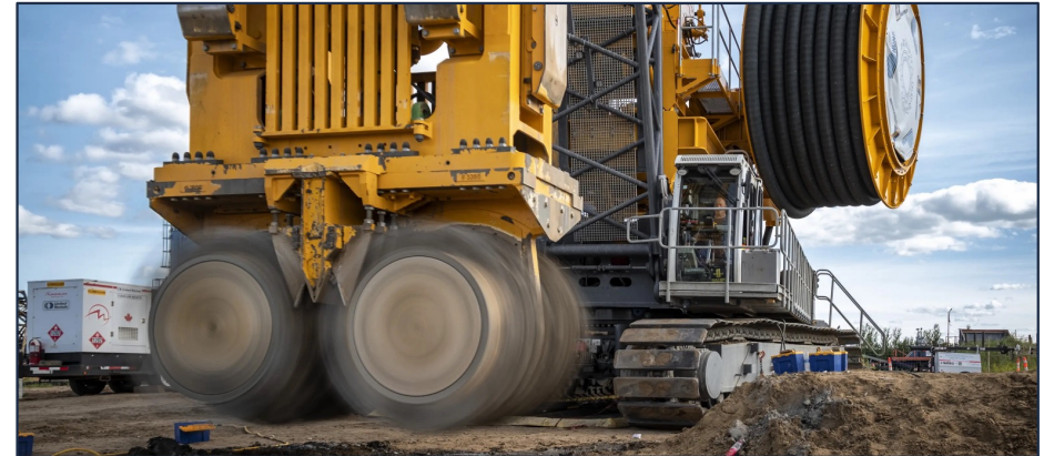
Diaphragm wall cutter with carrier unit in use on a construction site [3]
