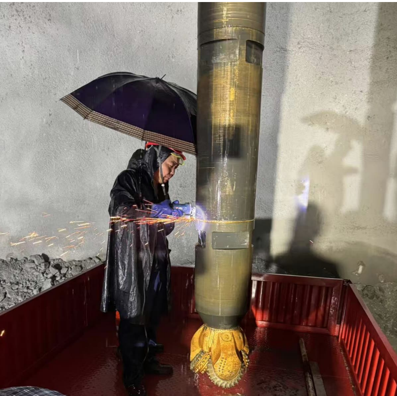
Pilot hole breakthrough
