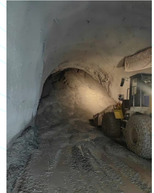
Muck discharge from bottom
