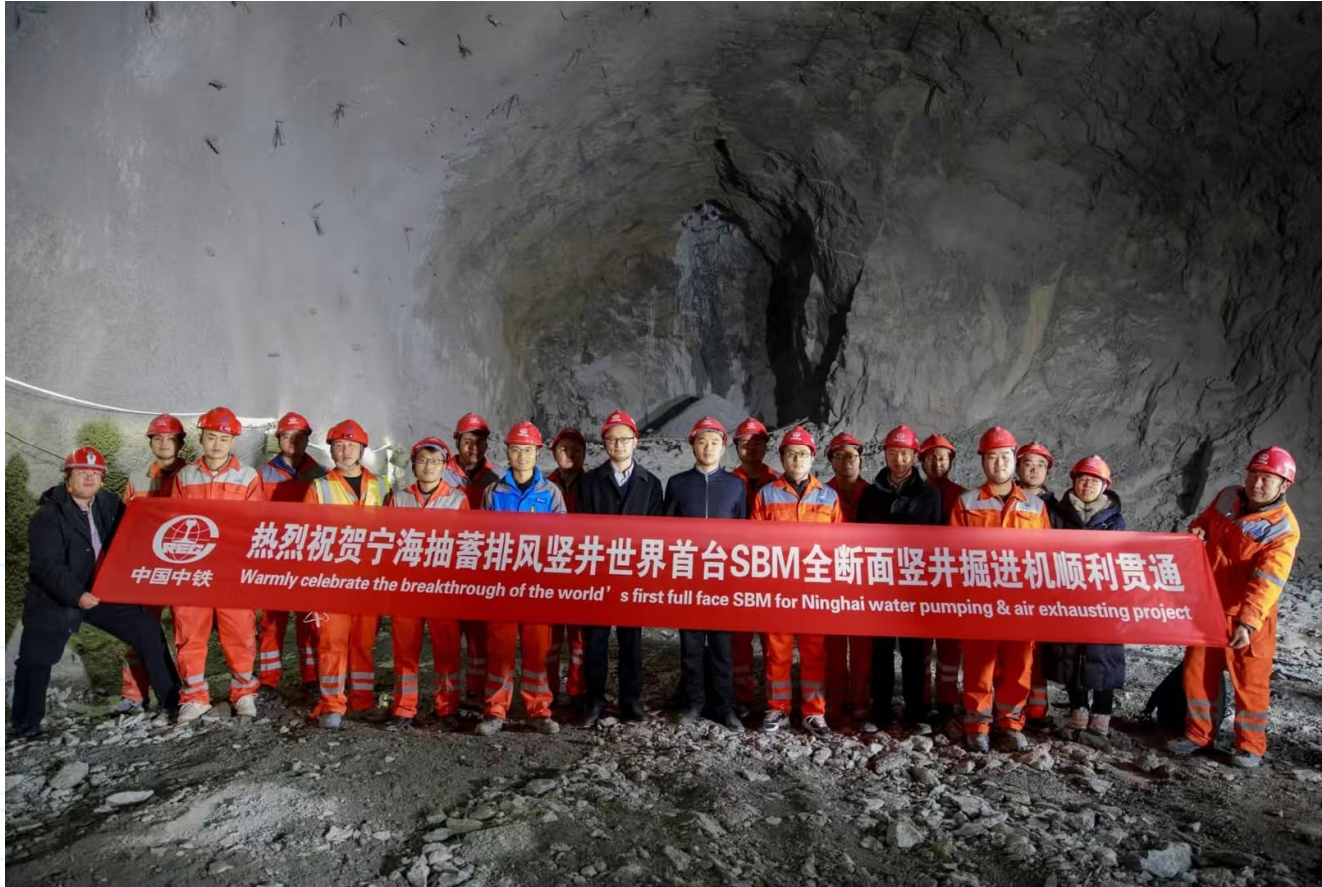
Ventilation shaft of the pumped storage power station
