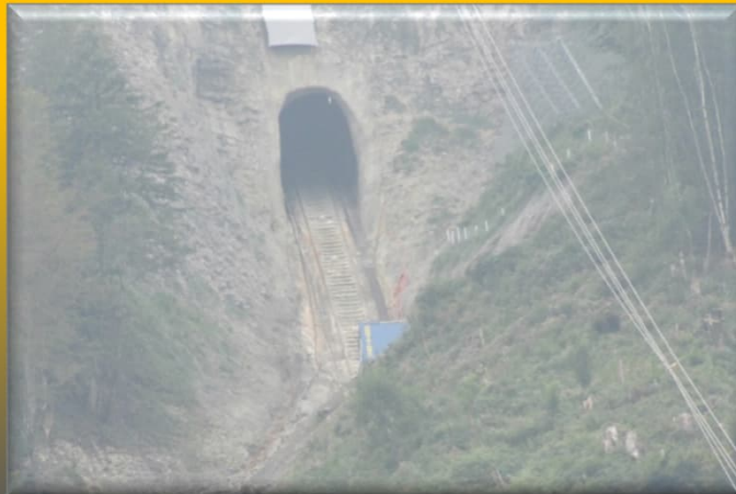
Pilot and Guiding Hole for Tunnel Excavation
