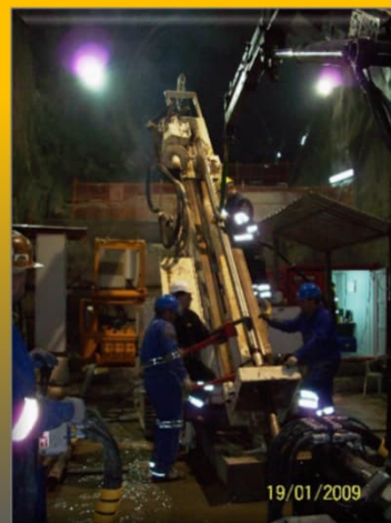
La Muela – Spain – Directional Pilot Holes for Hydropower Projects
