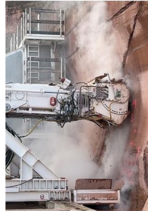
Roadheader excavation
