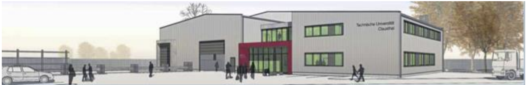
Drilling Simulator Celle
