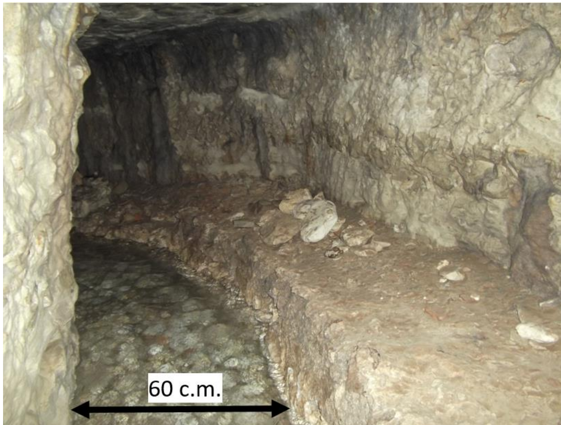
Figure 22: One tunnel at Harun spring S-8 (Photo taken by Raghid Sabri 2011)
