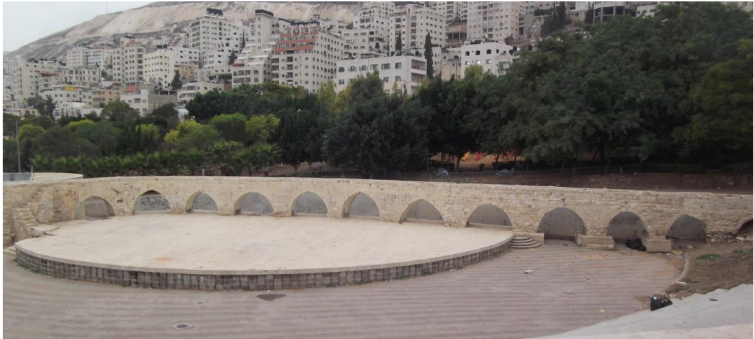
Figure 9: Nablus aqueduct from Islamic era (Pointed Arches) (Photo taken by Raghid Sabri 2011)
