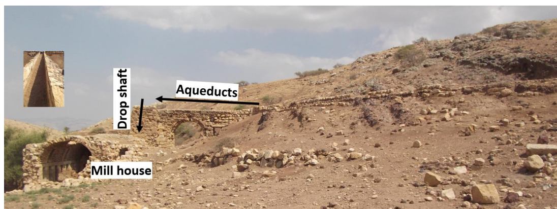
Figure 99: Arrows represent the water flow through the aqueduct and millhouse at Al Malih, top left: view to the aqueduct (Photo taken by Raghid Sabri 2011)
