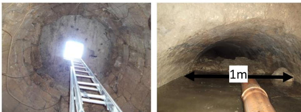
Figure 24: Carbonate sinter accumulated at the entrance of Harun spring tunnel S-8 (Photo taken by Raghid Sabri 2011)
