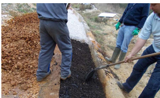
Fig. 8: Installing the passive AMD treatment channel
