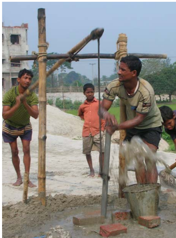
Fig. 4.1.1.2. Well construction by the local „hand flapping“ method
